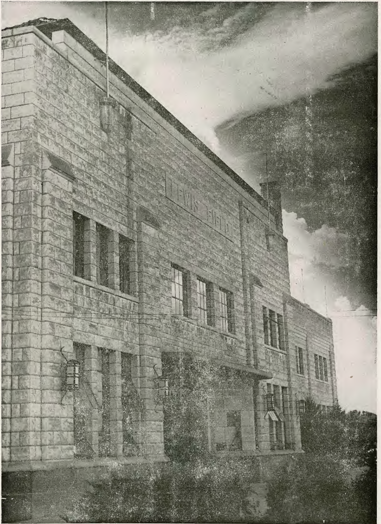
LEWIS FIELD STADIUM
